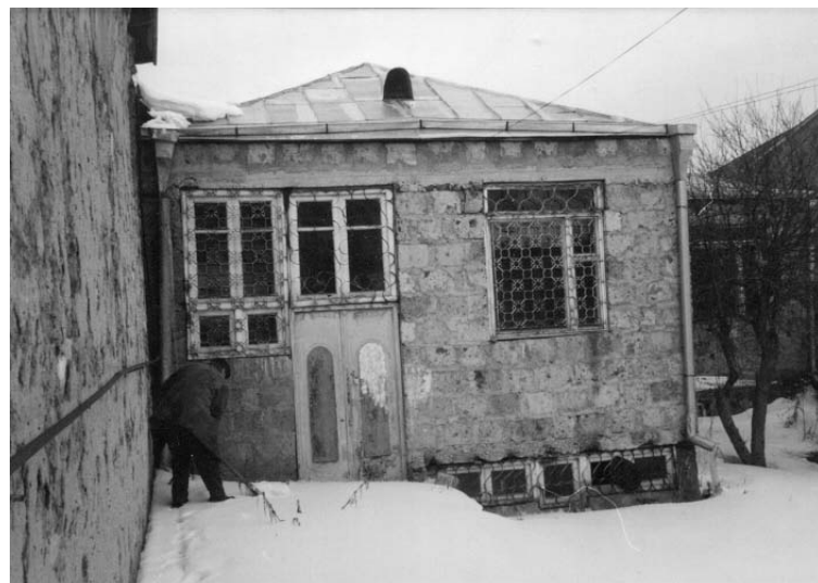
Gavar Satellite Clinic: an old house BEFORE the renovations
