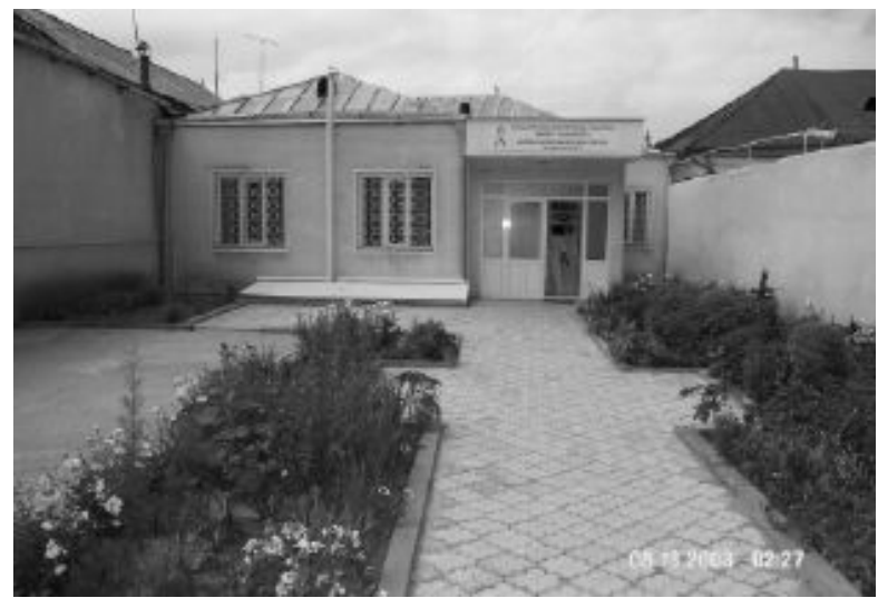
Gavar Satellite Clinic: NOW - after the renovations
